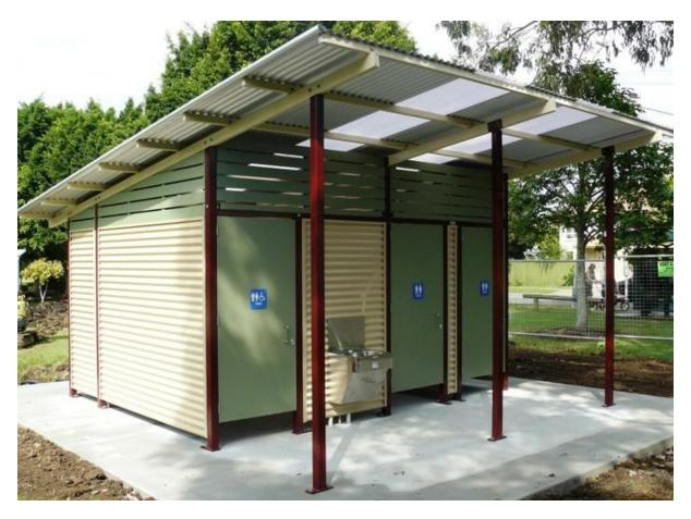
The Burley Restroom has four of the key CPTED features: sight lines under the doors and walls, external hand wash and water supply, space to take in a bicycle/pram/wheelchair etc. and robust construction. For more details see:
